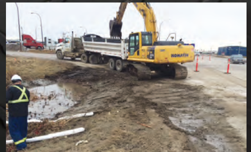
Spill site restoration
